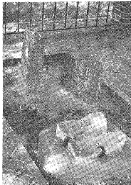
Figure 2. Base of vandalized Middle Point stone.
