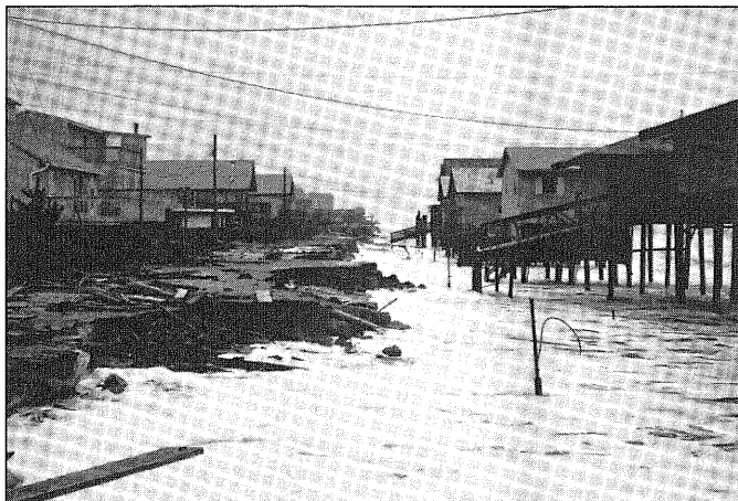
View of Ocean Drive in South Bethany showing damage caused by wave action.
