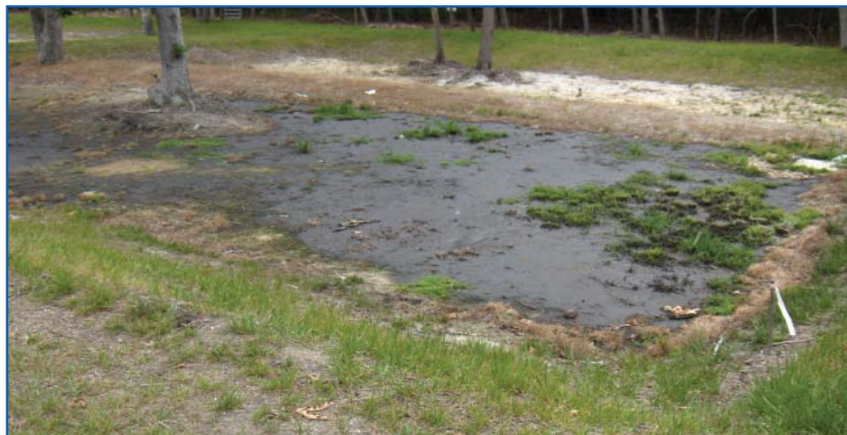
RIB at Southwood Acres (Kent County) with treated effluent during infiltration cycle.
