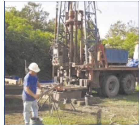
Driller Gene Cobbs III removing the shoe of the core barrel.
