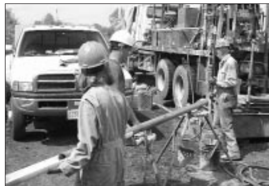
Extruding a 10-ft cored section. From left to right, Stefanie Baxter, Tom McKenna, and USGS driller Gene Cobbs.
